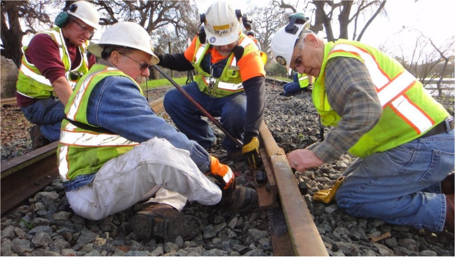
Mike H., Mike F., and Mike W. bolt the last stick into place
