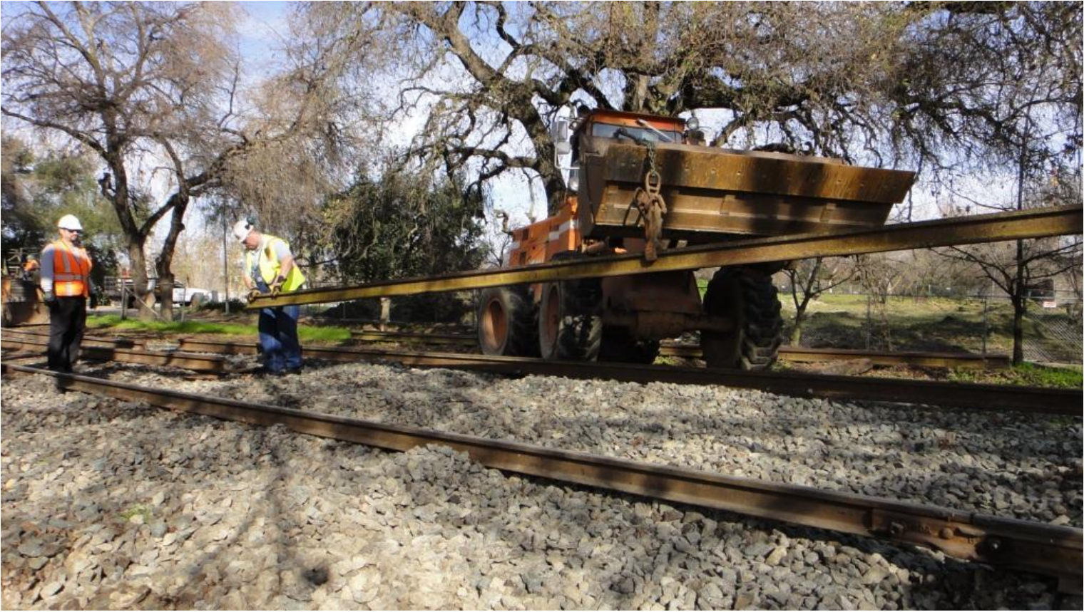
Chris guides the last stick of rail into place. Jose stands ready with the rail-saw as it needed to be cut in order to fit
