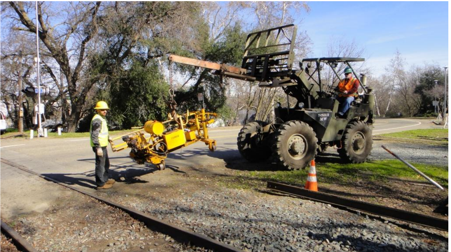
Chris M. guides the spike puller as Al on Big Green comes in to grab it off the track
