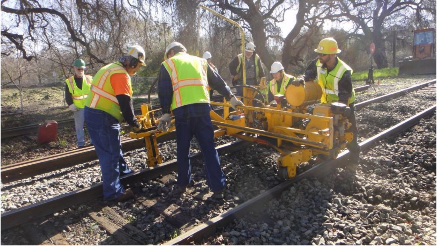
Mike F. gets the spike puller working but, Chris M. has to operate the throttle manually
