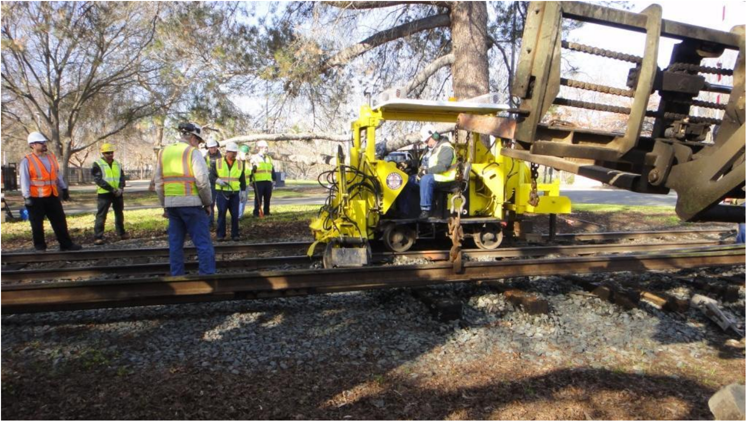
Al on Big Green lifts the assembled replacement rail so that Chris C. on the Jackson 125 can remove ties
