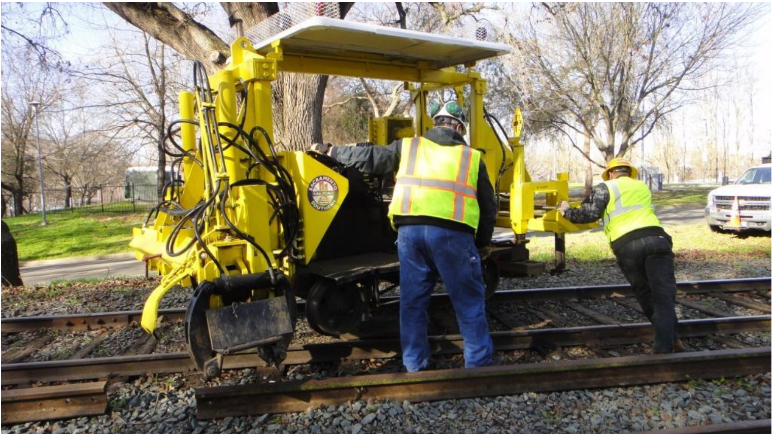
Spinning the 125: Chris C. and Chris M. spin the 125 so that it can start pulling ties to the west
