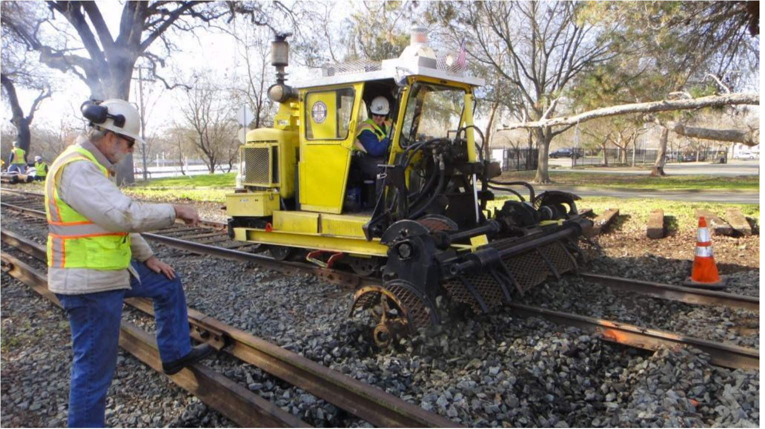
Heather in the scarifier digs out the tie-cribs under Alan's direction
