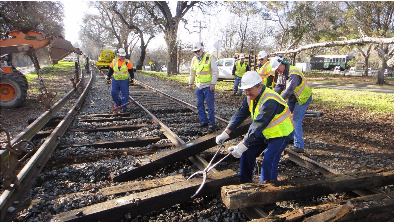
John and Steve move more dead ties out of the way
