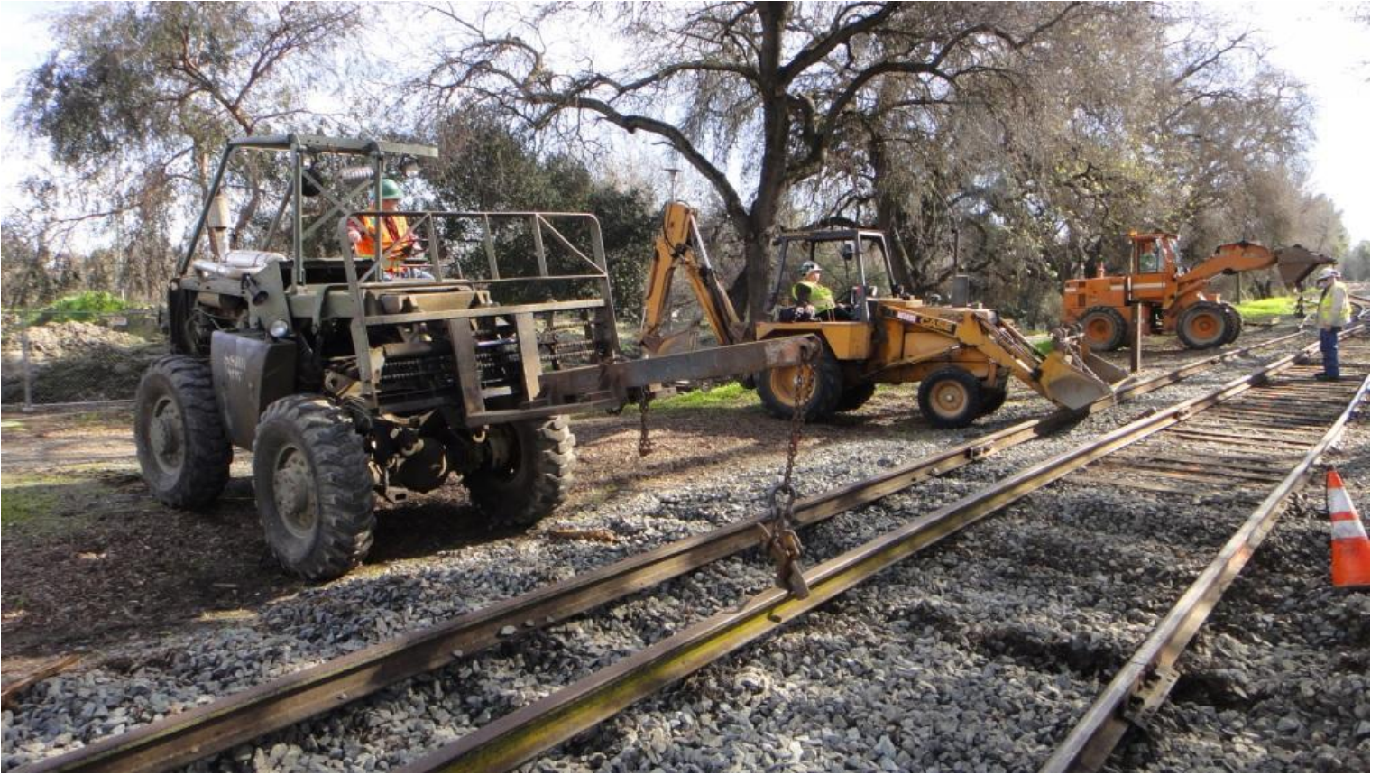
Ready? Set. 1, 2, 3 – GO! Alan directs Al on Big Green, Harry on the back-hoe, and Mike H. in the loader as they lift, in unison, the new east-rail into place
