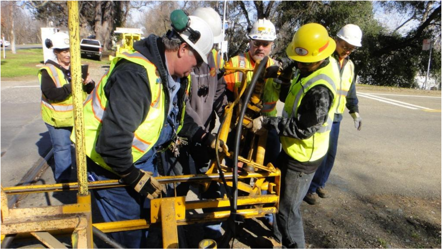
Deploying the spike-puller entails attaching the spike-pulling ram. It's a four-man job to move this awkward and heavy beast – a simple task for Chris C., Steve, Mike F., Chris M.
