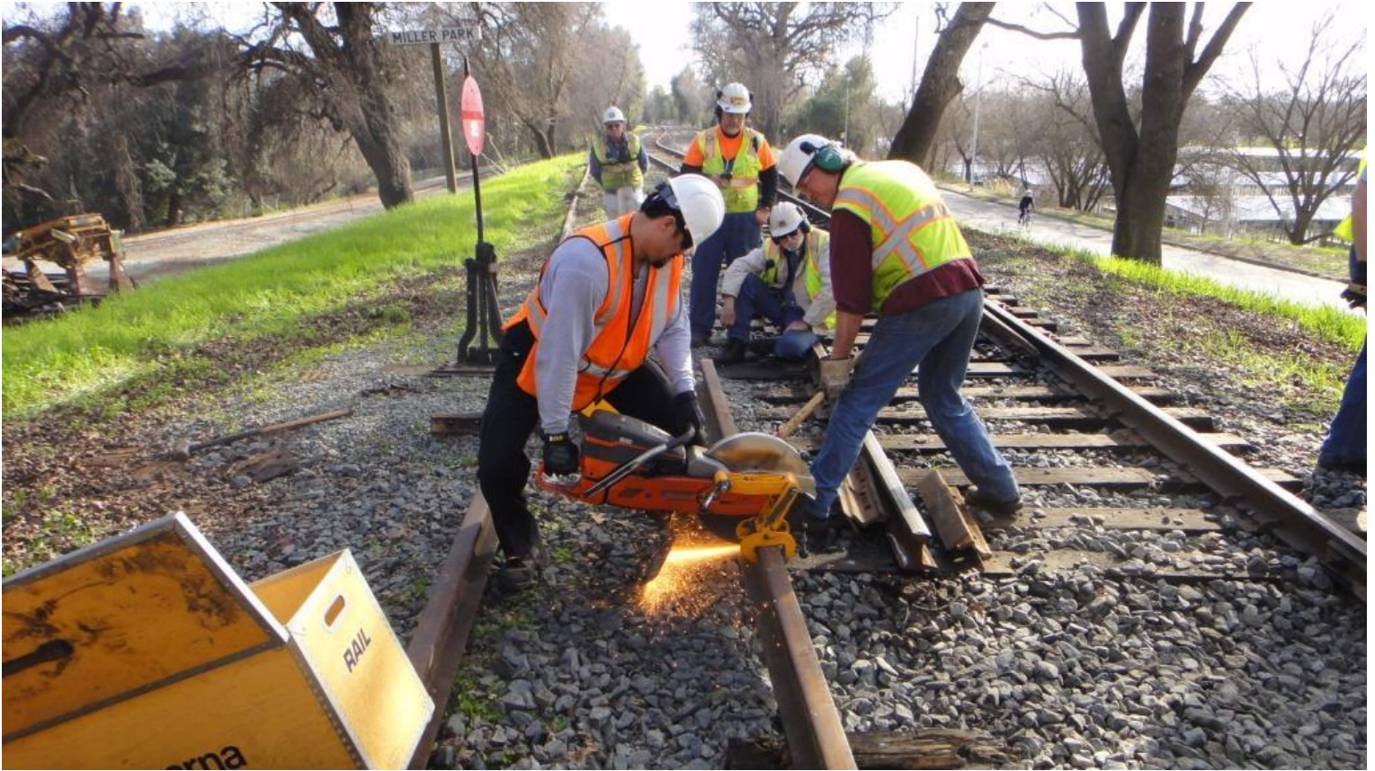
Jose deploys the rail-saw and Steve uses a shovel as a spark-shield
