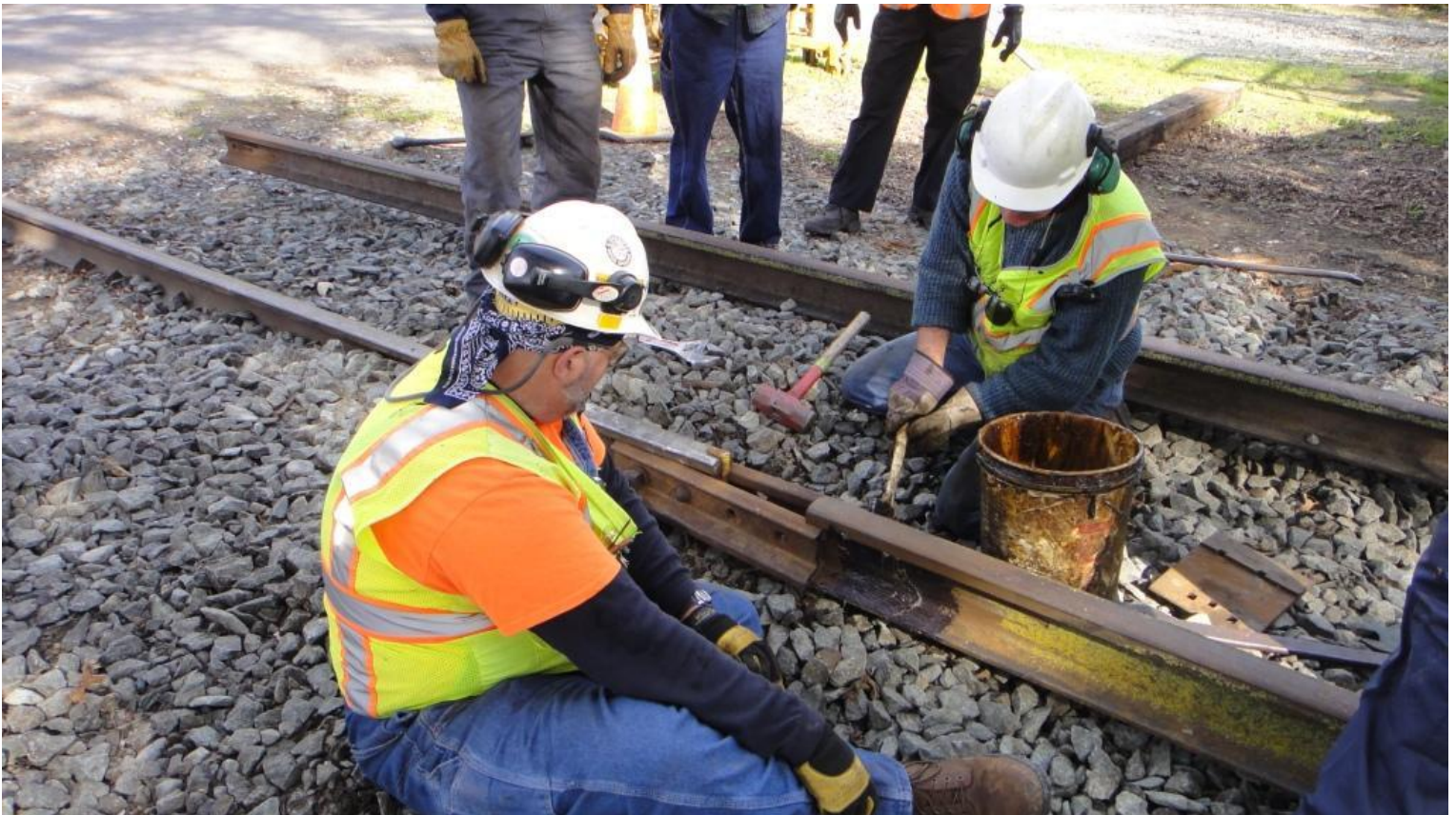
As the track heats up, it expands. So, Steve slathers grease on the rail-ends which will help the with thermal expansion within the joint
