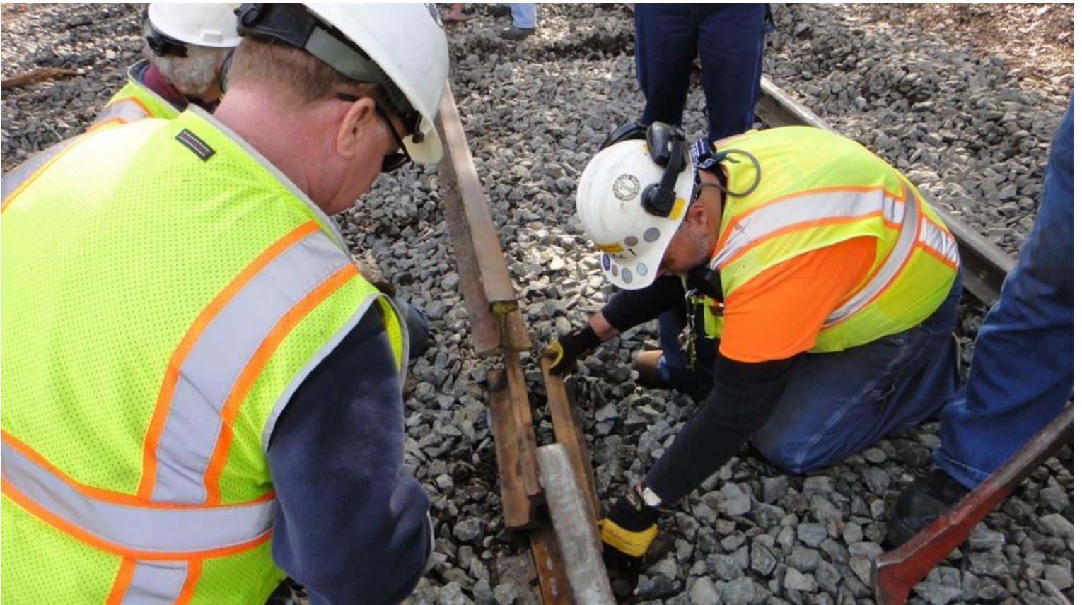
Steve, Ed, and Mike F. prepare joint-bars to attach the new rails up to the track
