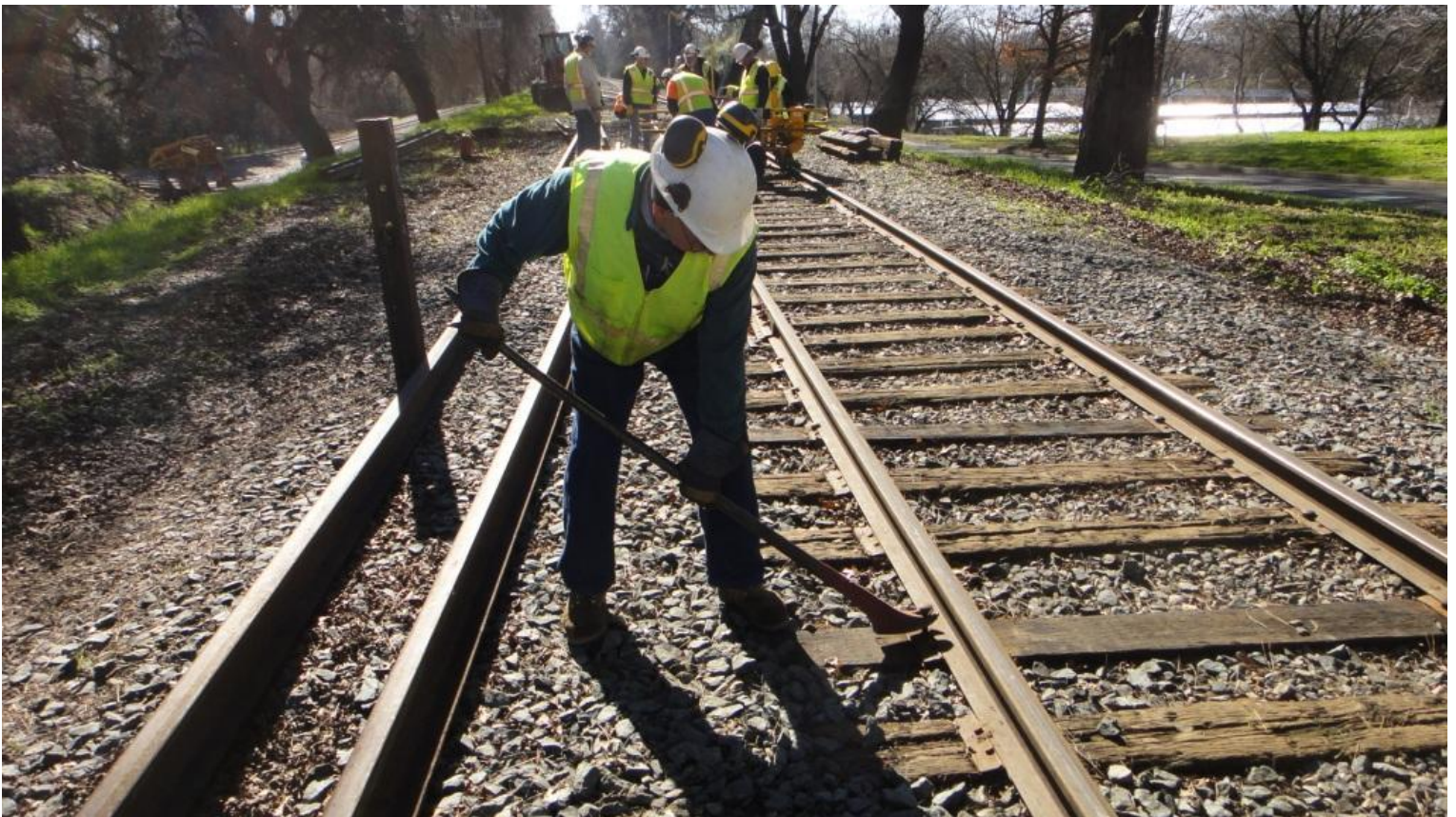
Meanwhile, Clem proves that man is mightier than machine and gets the spikes along the east-rail pulled...
