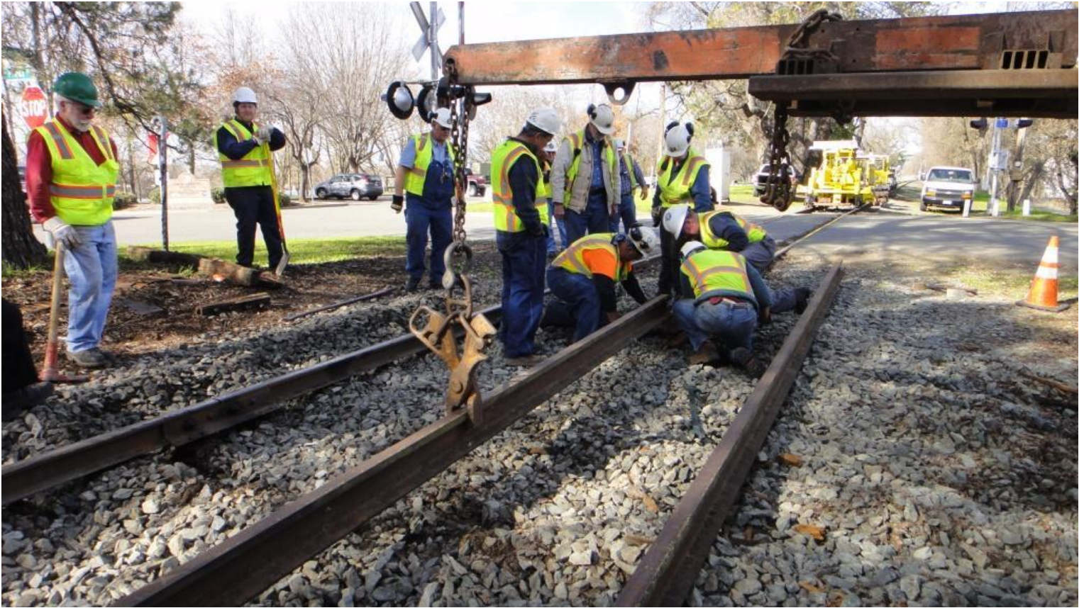
The "stinger" Big Green supports the new east rail as Mike F., Steve, and Ed line the rails up in order to bolt together
