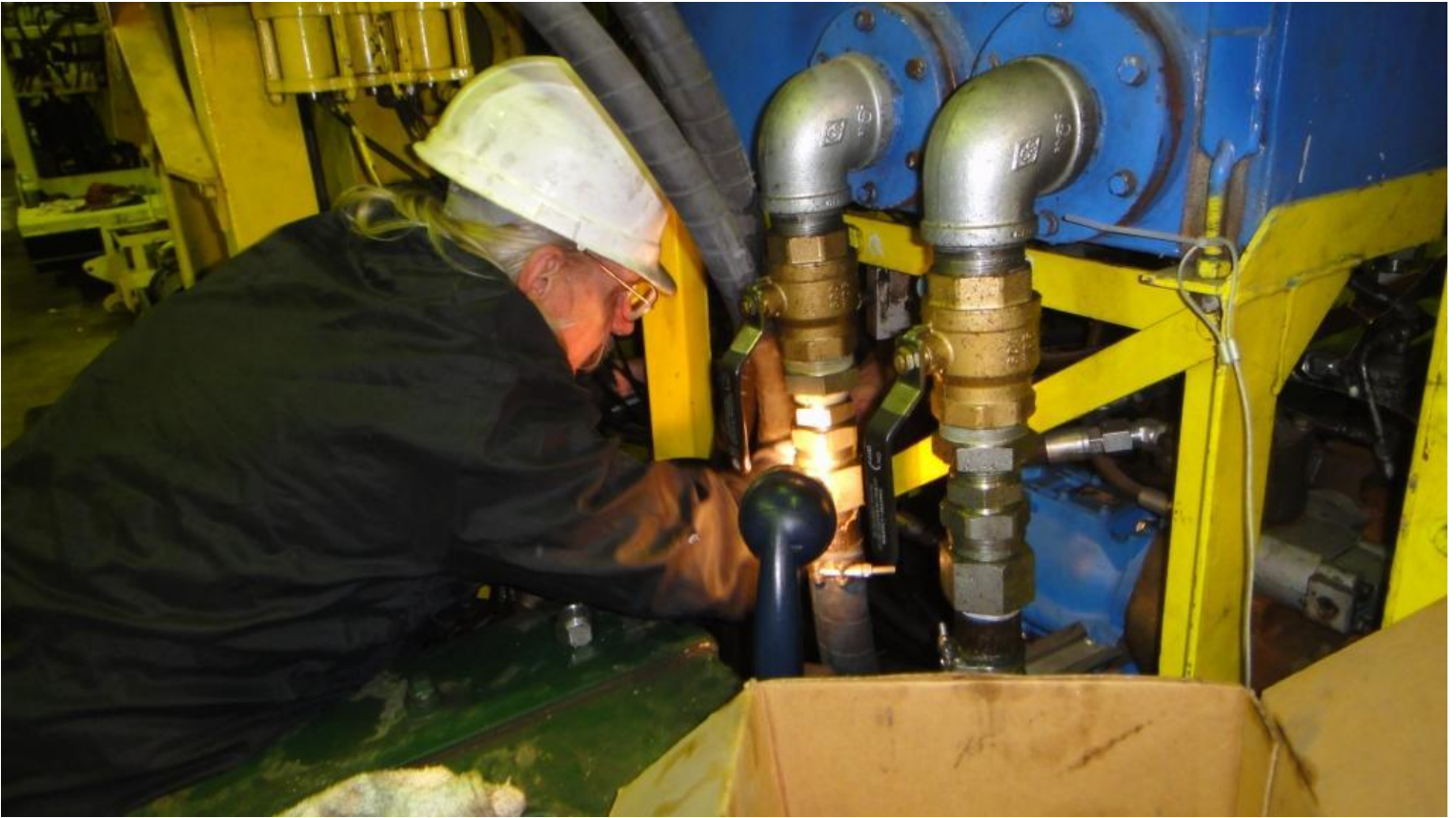
Fred installs the new hydraulic hoses on the tie-shear
