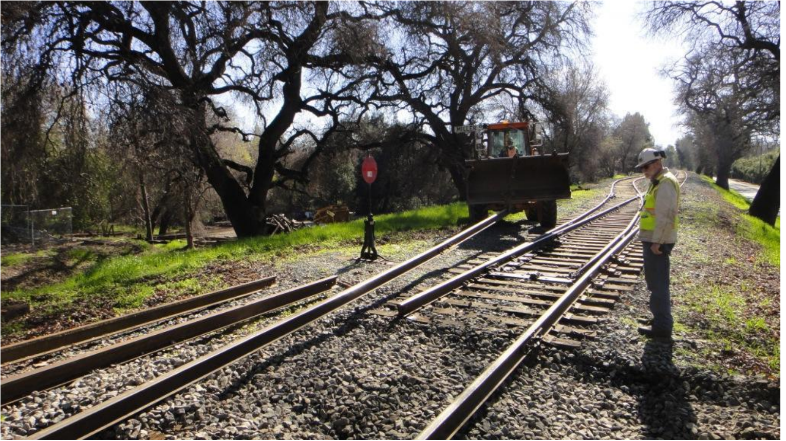
Mike H. in the loader removes the old east-rail
