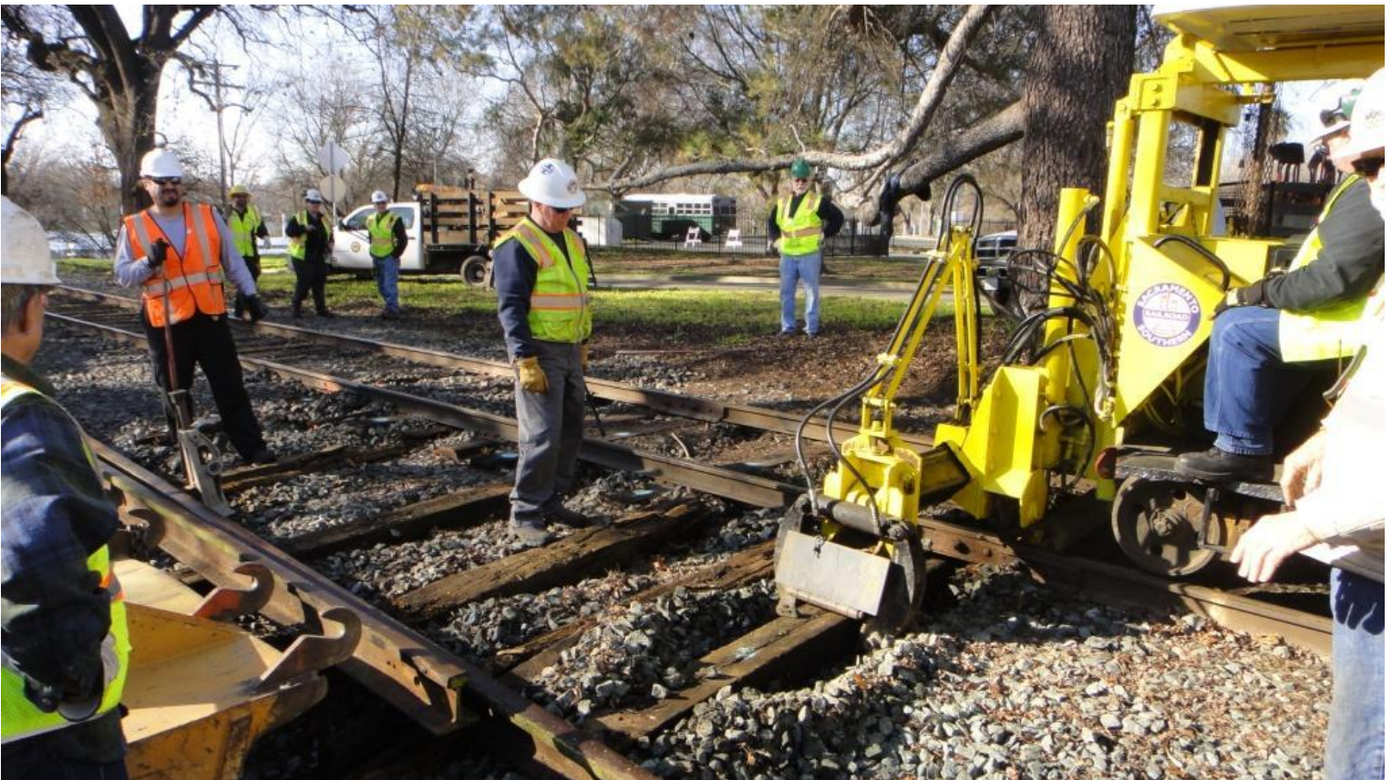
Ties at the north end being removed in order to lower the road-bed. The existing 75 lb. rail is 1¼ inches shorter than 110 lb. rail replacing it
