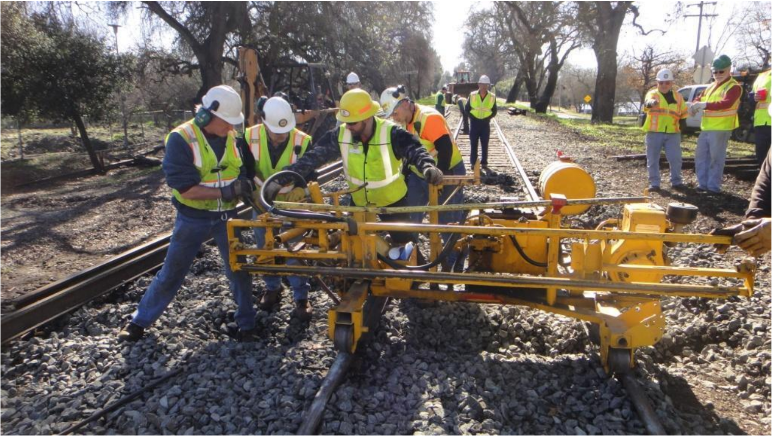
Because the joint has been taken apart and the rails out of alignment, Steve uses a lining bar to hold the rail in place so that Mike W. and Chris M. can move the spike-puller to a place where it can be removed from the track
