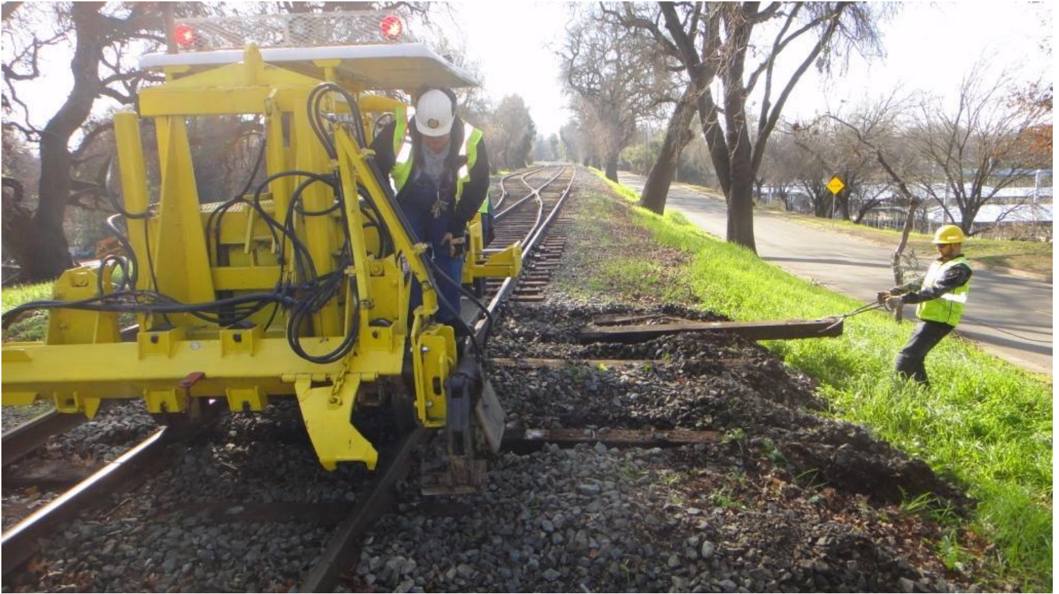
Chris C. on the 125 pulls ties out from under the track while Chris M. clears them out of the way
