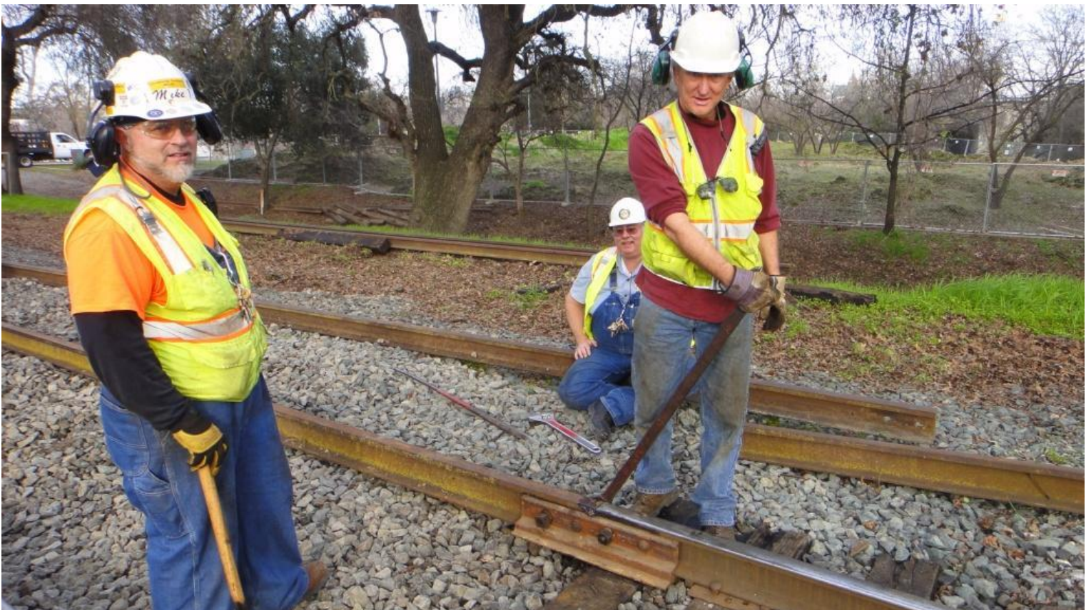
Steve tightens the last bolt at the comp-joint as the new east rail is attached to the south end
